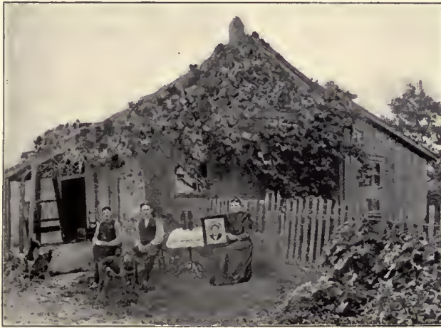
A DWELLING BUILT OF CLAY AND STRAW MIXED, IN THE SOUTH OF RICHLAND COUNTY. BUILT IN AN EARLY DAY AND USED UNTIL RECENTLY
